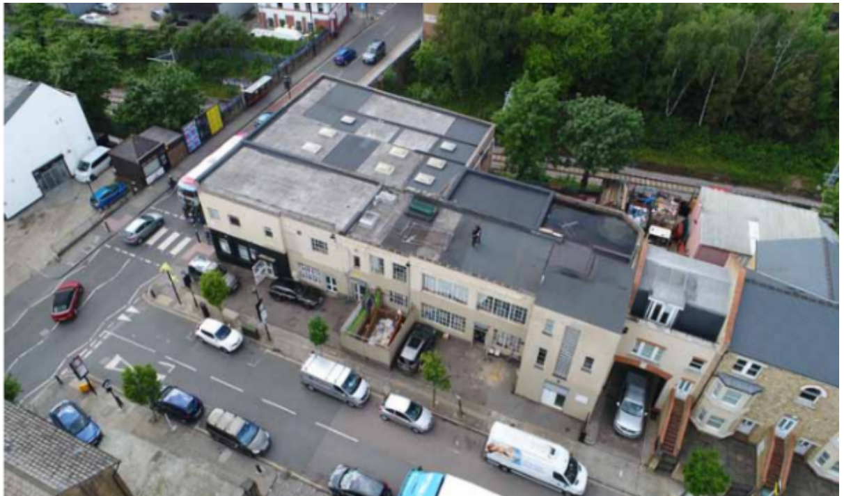
Aerial View of Grenville Road Elevation (North Site)
