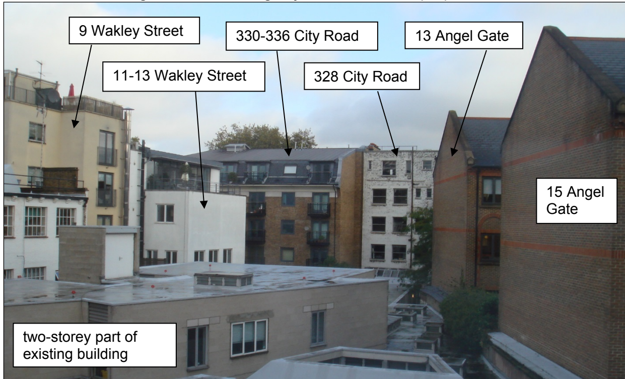
View north from Angel Gate indicating adjacent residential properties
