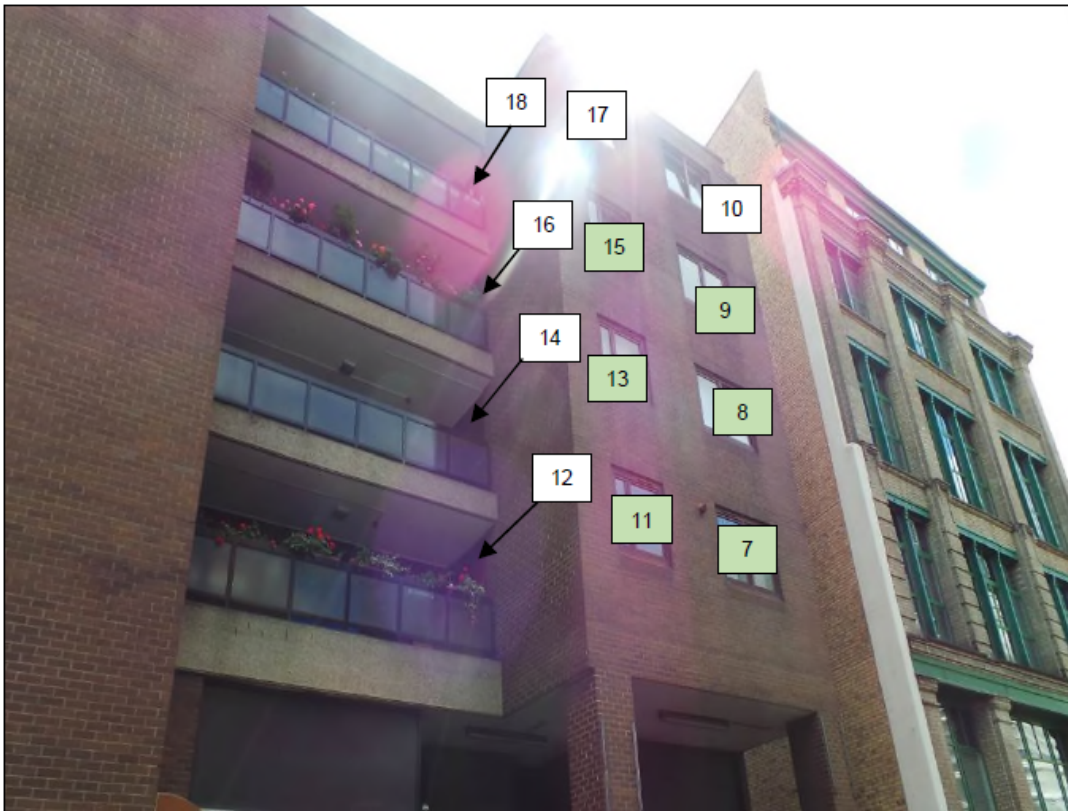
Figure 14: Assessed windows to the north west of 10 Epworth Street
